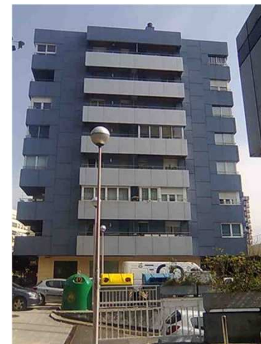
Existing building - Spain
